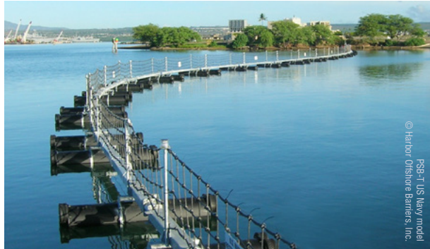
PSB-T completes waterside perimeter security.
