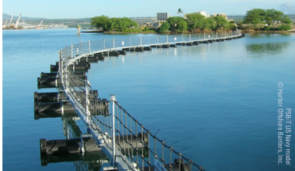
PSB-T completes waterside perimeter security.
